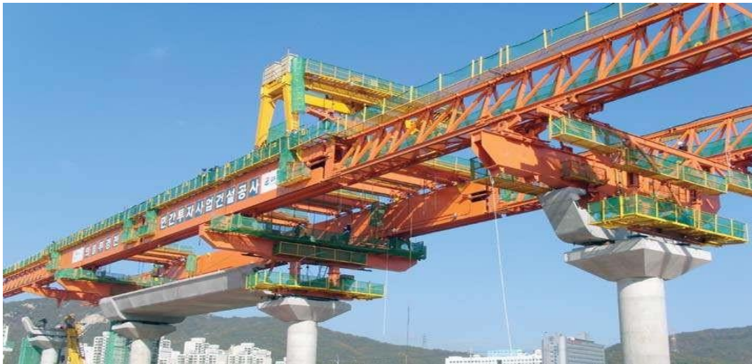
Long twin-upper-beam gantry is used for balanced-cantilever erection
